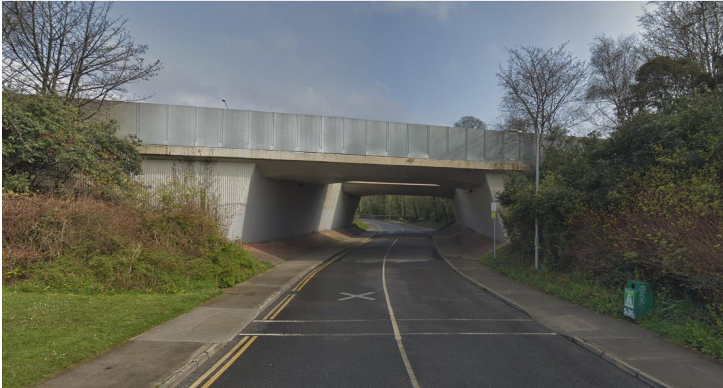
Figure 3: View of Existing Bridge (Southern Elevation)
